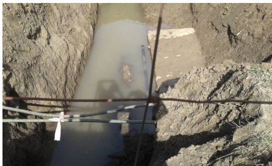
Fig. 4. View of construction site from the point of eligibility of maintenance and durability of pipelines and pipeline landfill resistance
