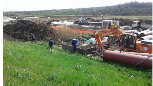
Fig. 2. View of construction site from the point of eligibility of maintenance and durability of pipelines and pipeline landfall resistance
