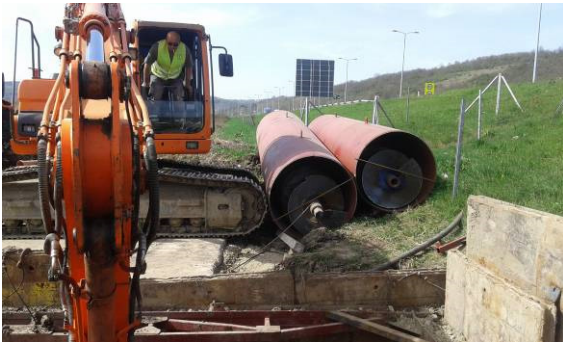
Fig. 3. View of construction site from the point of eligibility of maintenance and durability of pipelines and pipeline landfill resistance
