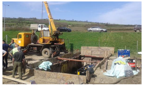
Fig. 7. Benefits during installation of ductile pipes
